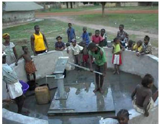
New borehole in Bafata
